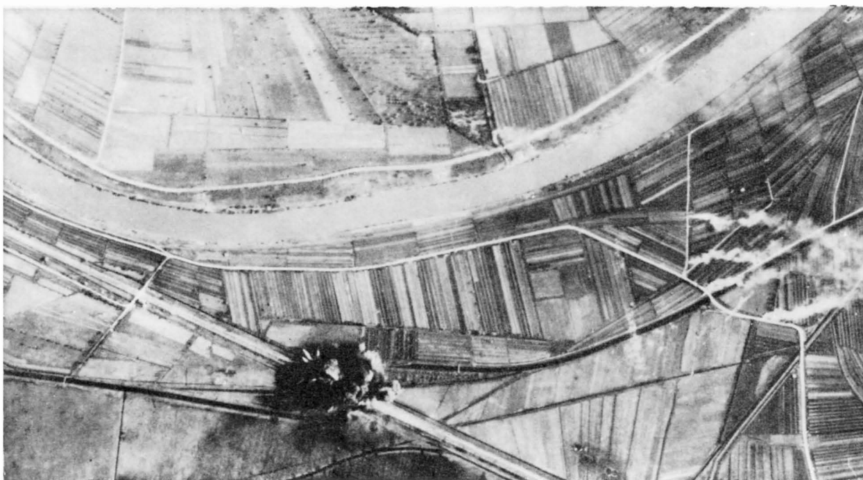
Both the span and abutment were destroyed by this excellent concentration of bombs on the small masonry railroad bridge north of San Michele.
