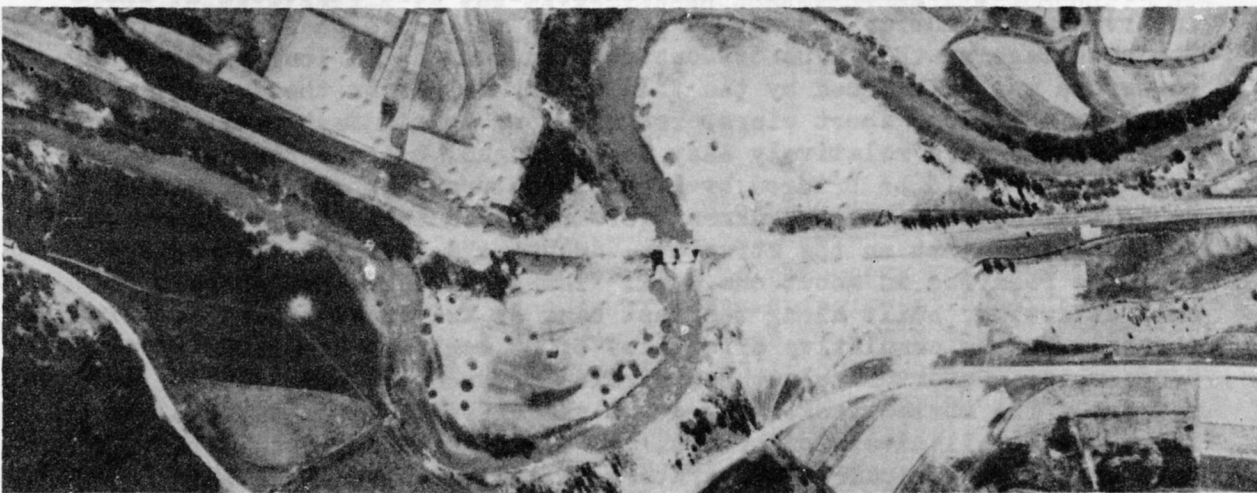
The top photo shows Campo rail bridge prior to attack by B-25s. The second photo shows the destroyed bridge the day after the successful attack on 21 April. The bottom photo shows the bridge repaired and passable nine days later. Repairs here were carried out by the typical construction of an intermediate pier and the laying of 60-foot repair spans.
